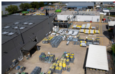
Oevel Plant in Belgium
